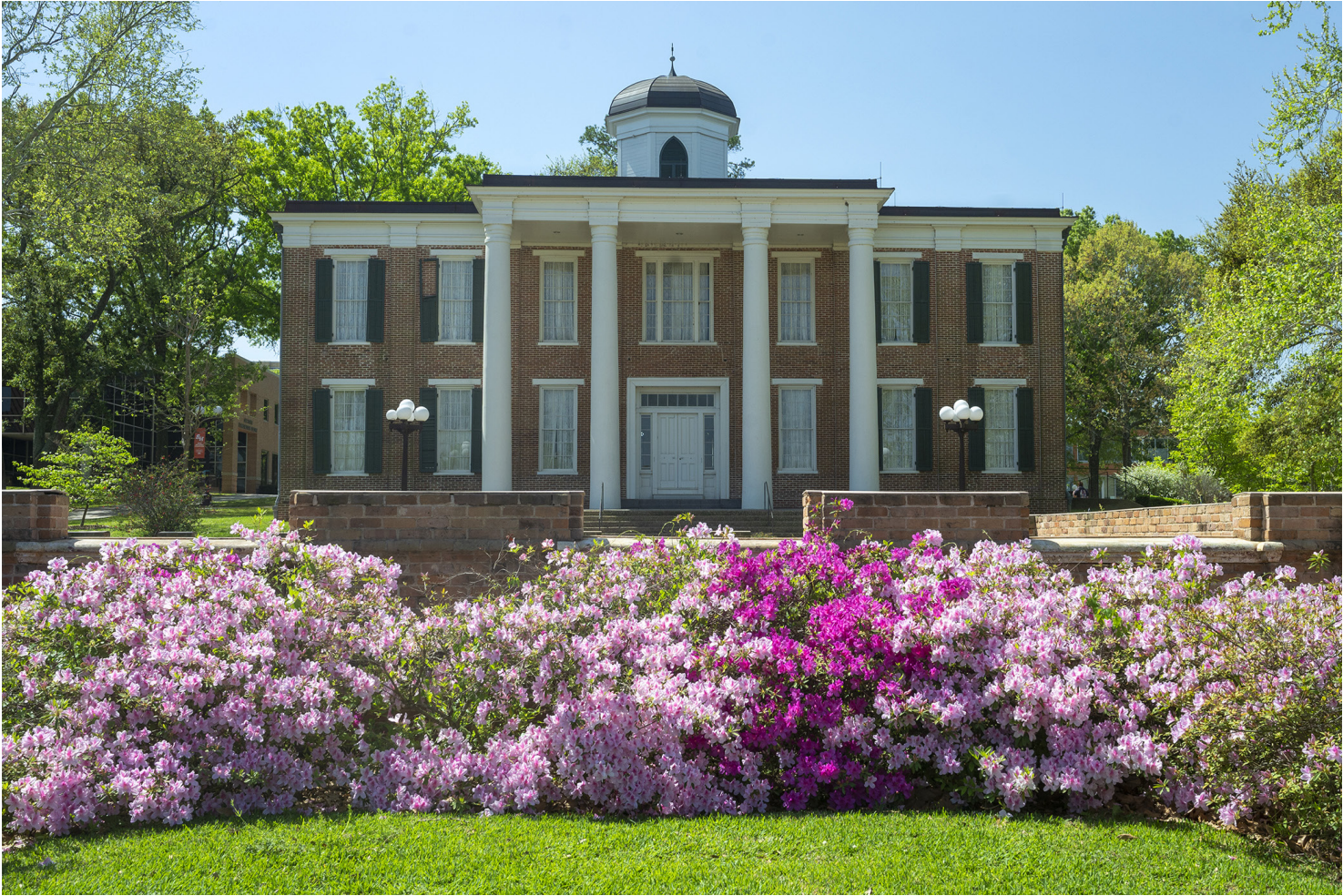
Figure 1.22 SHSU Historic and Contemporary Facilities
